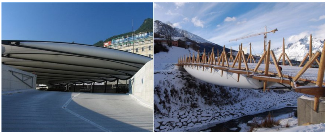
Fig. 2. Tensairity applications: Roof over a parking garage in Montreux with 28 m span (Luscher Architectes SA & Airlight Ltd, left) and a skier bridge with 52 m span in the French Alps (Charpente Concept SA, Barbeyer Architect & Airlight Ltd, right).
